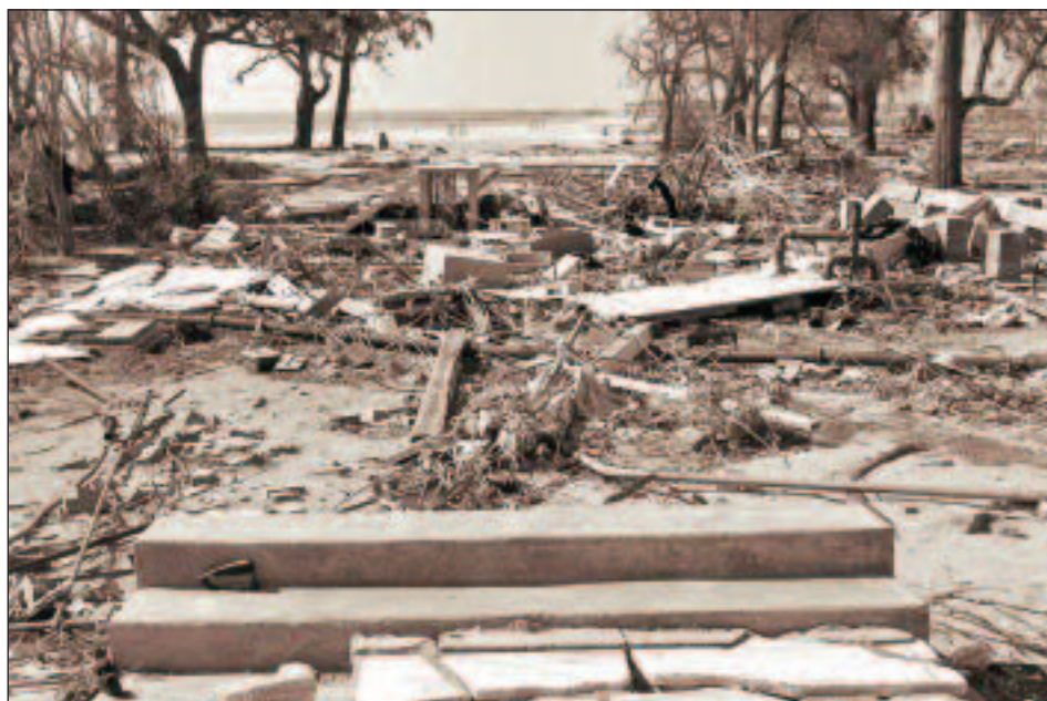
Damage from Hurricane Katrina to the law office of Boyce Holleman, PA.
